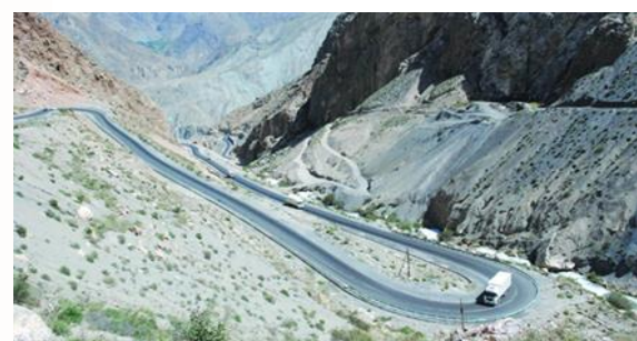
Dushanbe-Chanak Highway, Tajikistan built by the China Road and Bridge Corporation (CRBC).
